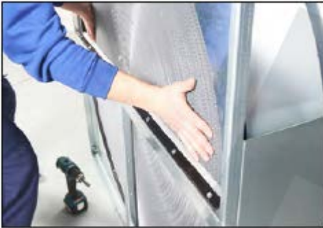
Figure 2 Carefully tilt the rotor. Ensure that the disc lamellas are not damaged.
